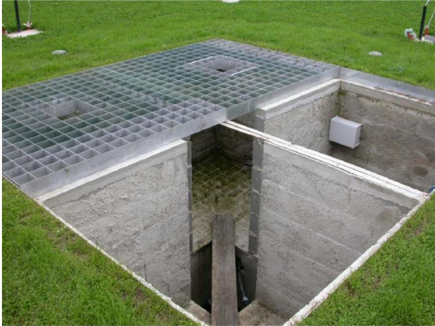
**Fig. 4:** The gratings, the pit internal walls and the pit recess for drainage (Vigna di Valle, Italy, 2007).
